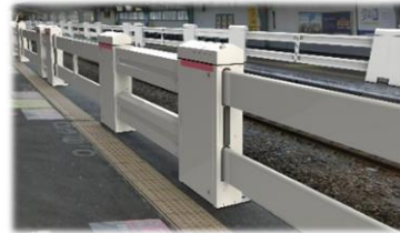
Moveable platform gates
